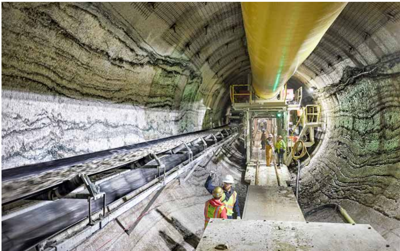
An overview of the extensive Robbins conveyor system for the DigIndy tunnels below Indianapolis, IN. Photo courtesy of Robbins.
